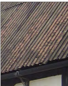
Modern sheet metal roofing
