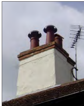
Rendered chimney stack
