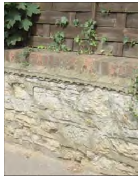
Rubble stone boundary walls, these are found in coursed and rough forms
