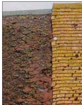
Fish scale roof tiles on Church Farm
