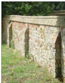
Brick buttresses are unusual but examples can be found on Stratford Road
