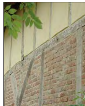
Plain and rendered brick infill panels to timber frame
