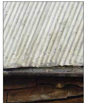
Modern sheet metal roofing
