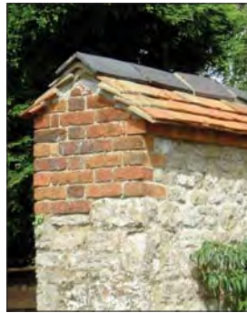
Rubble stone boundary walls, these are found in coursed and rough forms
