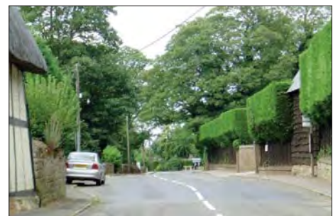
View looking west along Stratford Road
