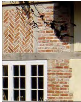
Herringbone brickwork at Wood End
