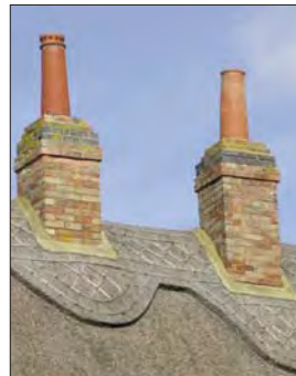
Tall terracotta chimney pots are common in Nash village
