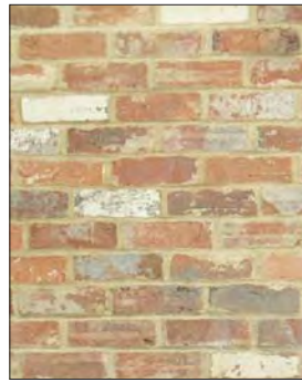
Stretcher bond - this brickwork was originally painted
