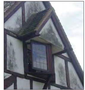
Unusual projecting first floor window on gable end
