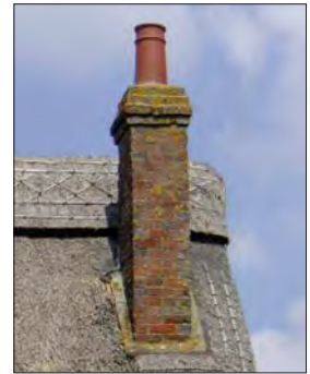
Brick gable end stack
