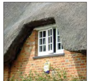
Thatch dormers at eaves height
