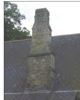
Rubble stone chimney on the Village Hall
