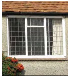
Unusual C20th leaded lights at Church Farm
