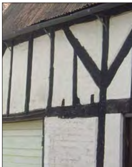
Painted brick infill panels to traditional timber frame
