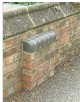
Brick buttresses are unusual but examples can be found on Stratford Road
