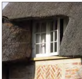
Thatch dormers at eaves height
