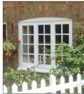
Traditional Victorian casement with arched brick header
