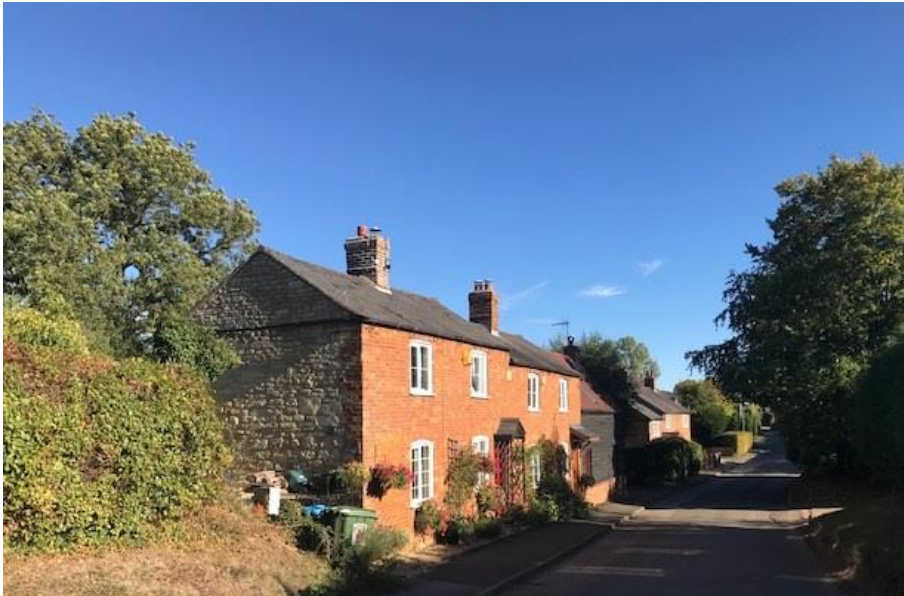
High Street, Nash, looking south, September 2018
